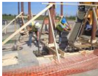
Port of Stephens City, VA. Radiation portal monitor foundation formation.
