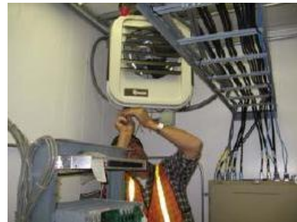
Biorka Island, AK. Doppler radar facility HVAC replacement.
