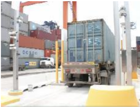
Port of Balboa, Panama. Ahtna-installed vehicle Radiation Portal Monitors and Optical Character Recognition cameras.
