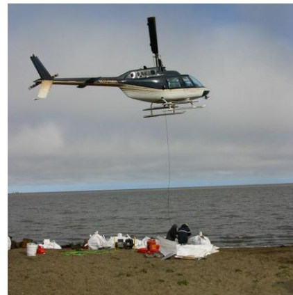
Pt. McIntyre, AK. A small crew was mobilized via helicopter to remove waste and debris.
